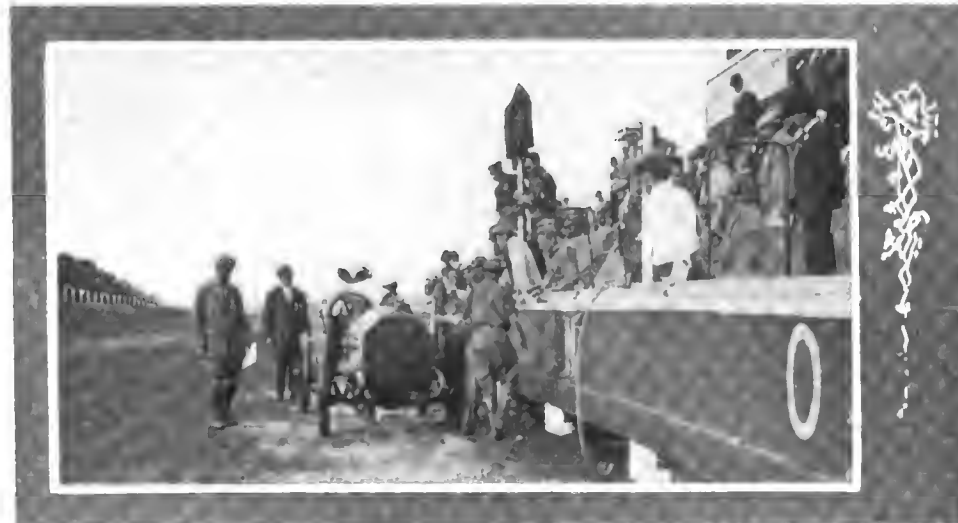
Especially Well Equipped Were the Pits for Rapid Work
